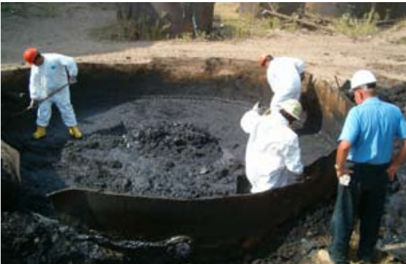
By 2006, the cleanup was underway. Here workers for the US EPA remove creosote in old tanks, reducing the potential for recontaminating cleanup areas in the river bottom.
